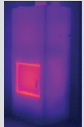
3 hour after heating Average surface temperature 37 °C
